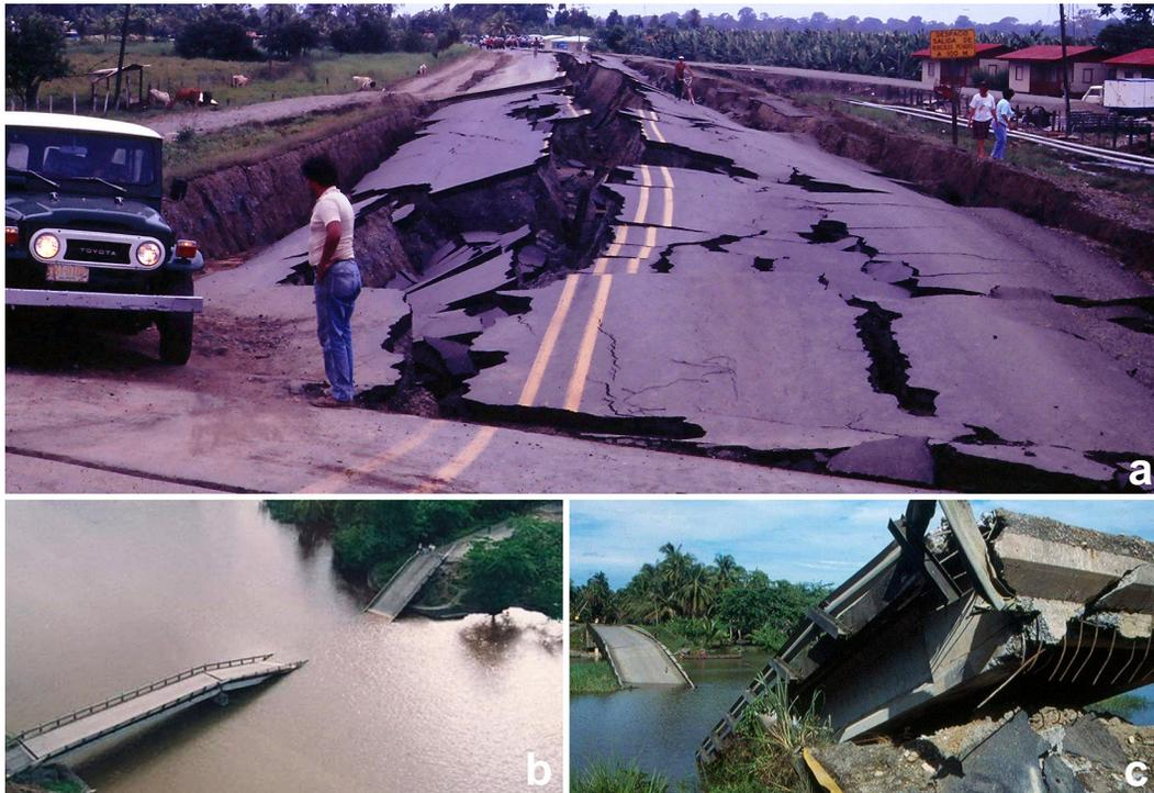
Fig. 5: Roads and bridges collapsed due to fracturing, lateral displacement and liquefaction. A destroyed road section close to Limón (a), and La Estrella river bridge (b,c). Photos provided by Sergio Mora Castro.
